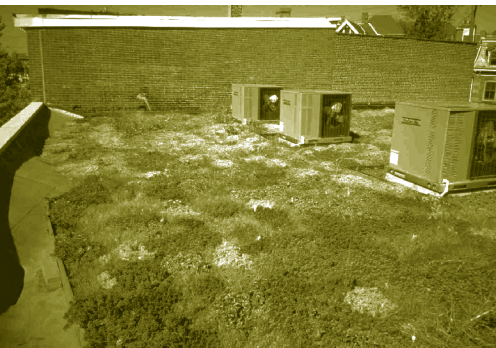
Above, top: The Ford Dearborn Truck Assembly Plant in Dearborn Michigan has a 10-acre green roof that is a 2004 Green Roof Awards of Excellence Winner. Photo: William McDonough + Partners
