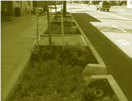
Above: Periodic curb cuts in an urban setting allow for streetside infiltration. Photo: Lower Columbia River Estuary Partnership
