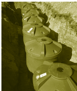
Above, top: The SmartStorm Rainwater Recovery System, developed by the Charles River Watershed Association; the cisterns and pumps can be easily hidden by landscape plantings. Photo: Charles River Watershed Association.
