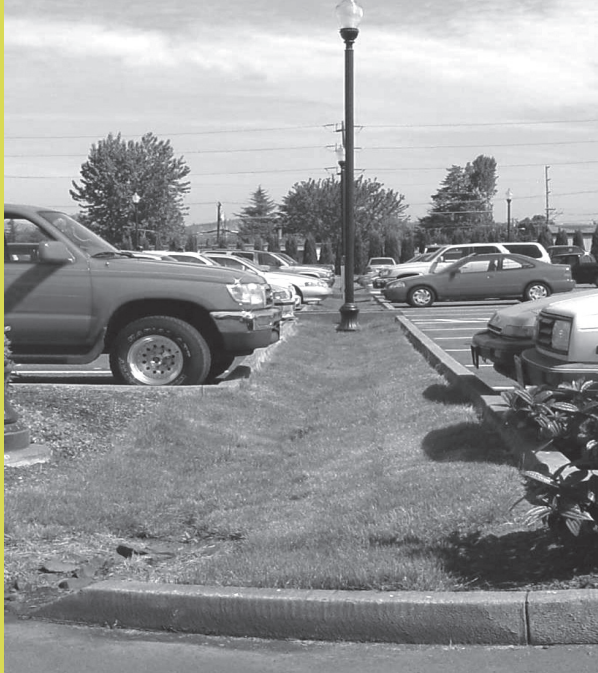
Above: Swales can be used on commercial sites to convey runoff around the site and to help slow peak discharge rates. Photo: Lower Columbia River Estuary Partnership
