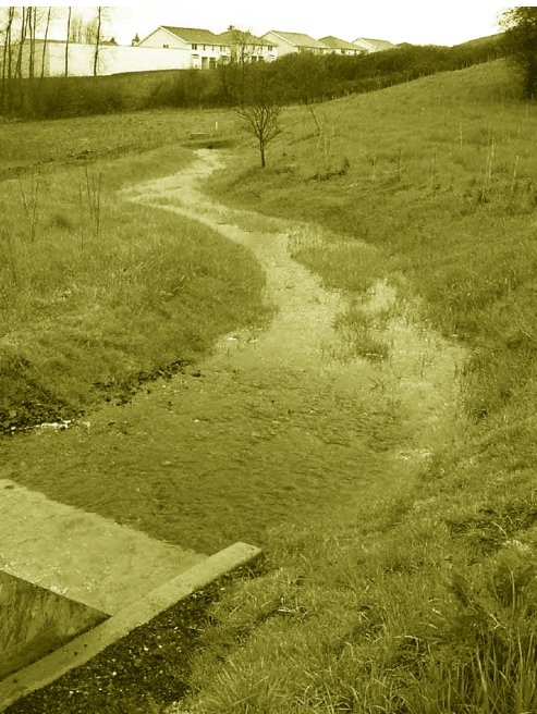
Below: A meandering grassed swale filters runoff and helps to improve site landscaping. Photo: Low Impact Development Center.
